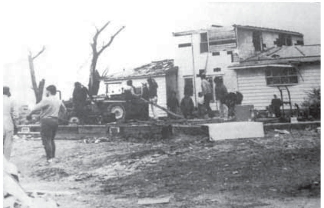
Volunteers clean up around the home of Larry Flickinger near Burrton in the days following the tornado.
